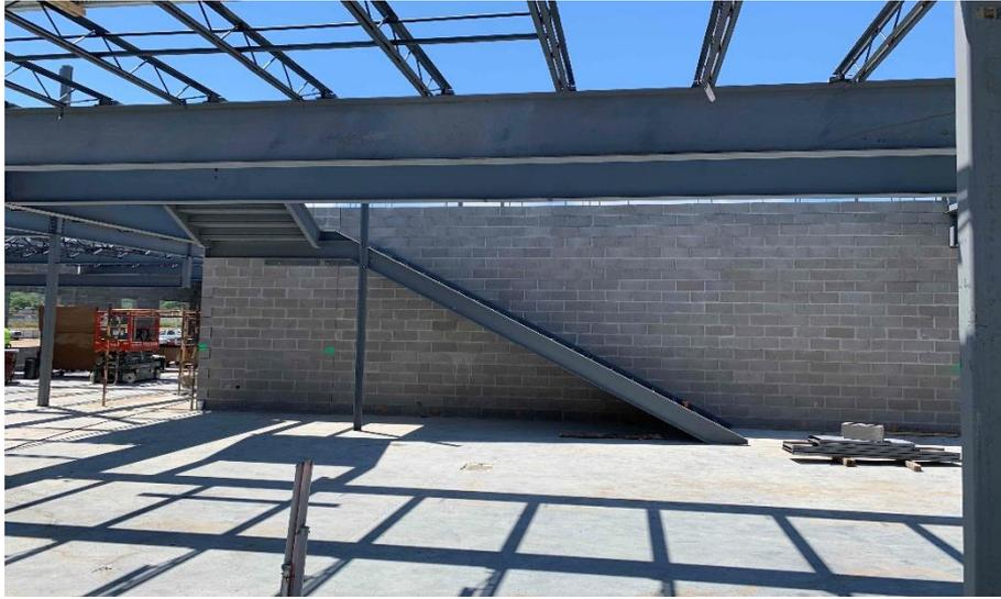
**Miami Whitewater Elementary:** The gym bearing walls continue to rise in Area A. In Area B, metal stairs have been installed up to the 2<sup>nd</sup> floor and layout has begun for the 1<sup>st</sup> floor interior walls. The North half of the 2<sup>nd</sup> floor steel is being set. In-wall and above ceiling MEP rough-in continues in both Areas.
