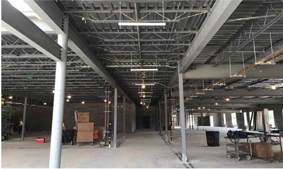
**Crosby Elementary:** In Area A, the stage bearing walls continue to rise and the mezzanine concrete floor has been poured. The steel joists in the gym are being detailed in preparation for roof decking. In Area B, the 1<sup>st</sup> floor interior walls and door frames are being framed and set. In-wall and above ceiling MEP rough-in continues in both Areas.
