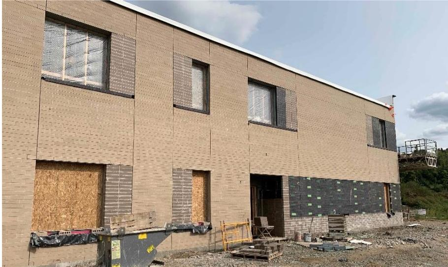
**Crosby Elementary:** In Area B, drywall is being hung on the 1<sup>st</sup> floor and interior CMU block walls are being laid around the restrooms on the 2<sup>nd</sup> floor. In Area A, the kitchen roof is being installed and steel is being erected in the administration area. Brick is being laid on the North and East wall of Area B. In-wall and above ceiling MEP rough-in continues in both Areas.
