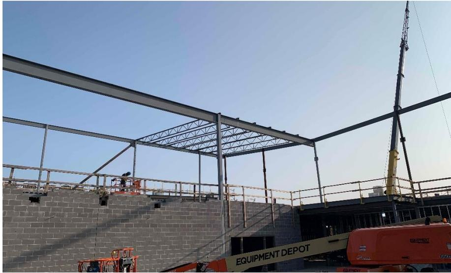
**Harrison Junior High:** Interior walls on level 2 of Area A and level 1 of Area B are being laid out and framed. Bearing block walls continue to rise in all three Areas while roof steel is being set on the 2<sup>nd</sup> floor of Area B. The concrete seating for outdoor classes has been poured in the courtyard. In-wall and above ceiling MEP rough-in continues in all Areas.
