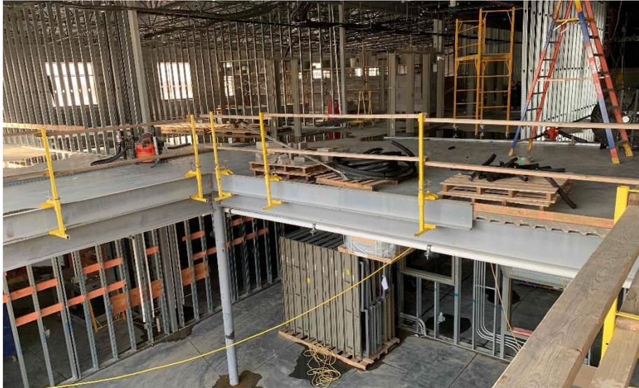
**Miami Whitewater Elementary:** Metal roof decking is being installed in the kitchen, mechanical, administration, and art room. In Area B, roof installation continues as the interior walls on the 2<sup>nd</sup> floor are being laid out and framed. Brick has begun on the East wall of Area B. Above ceiling MEP rough-in continues in both Areas.
